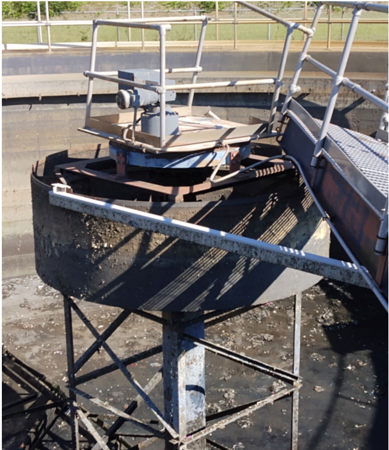
Photo #1 - Failed Sludge Thickening Equipment (Basin No. 2) Wastewater Treatment Plant City of Natchitoches, Louisiana
