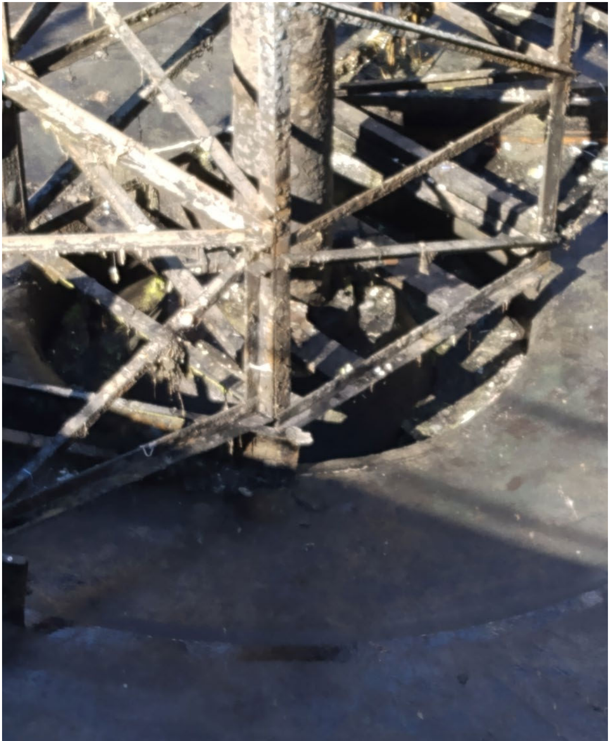
Photo #3 - Failed Sludge Thickening Equipment (Basin No. 2) Wastewater Treatment Plant City of Natchitoches, Louisiana
